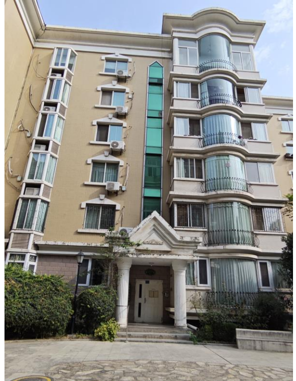
figure 46 Photo I take in new residence I am living now, 2025
