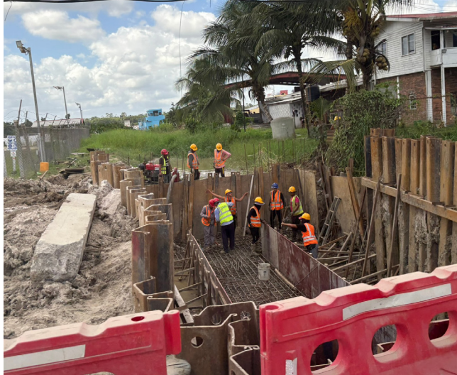
Construction workers in the midst of improving and expanding the road and irrigation infrastructure in Georgetown, Guyana. (Photo credit: Correia-Damude, 2026).
