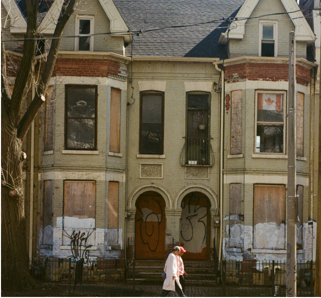
A boarded up building that was once affordable housing in Toronto. Now set to be re-developed into a higher rent condominium. (Photo credit: Correia-Damude, 2026).
