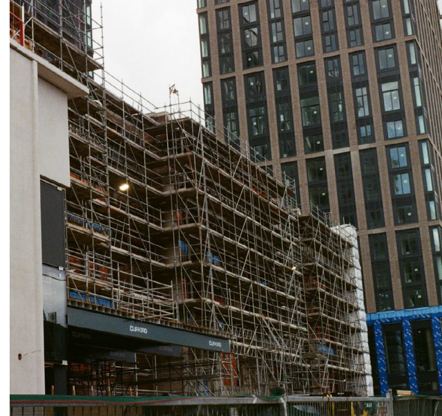
Toronto continues to develop and expand with aspirations of meeting the needs of its residents. (Photo credit: Correia-Damude, 2026).
