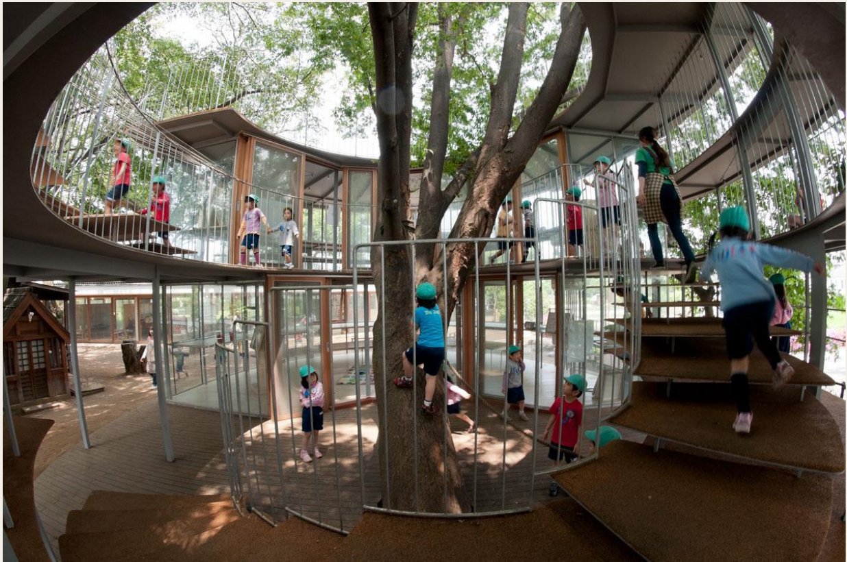
Rhythmic timber structure supporting visual coherence (Tezuka Architects).
