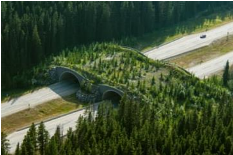
Figure 9: An overpass in a highway
