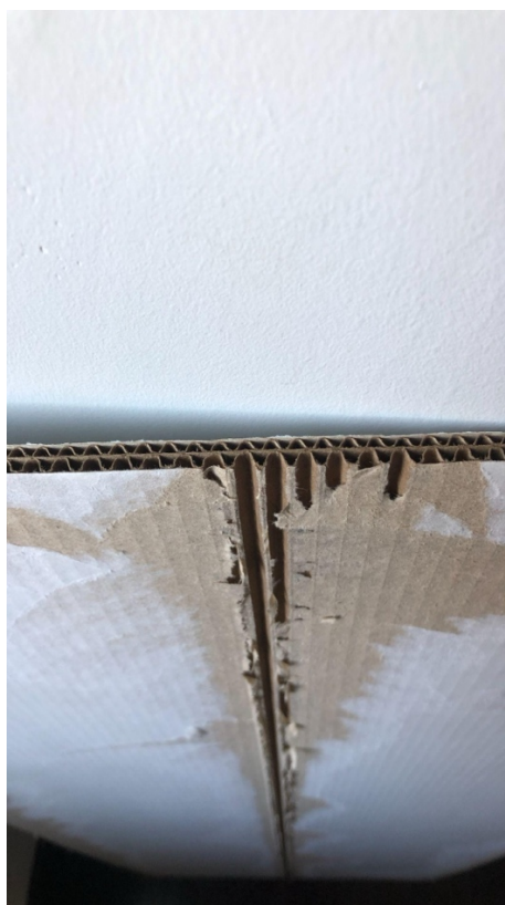
Figure 4. Early stages of preparing the substrate
