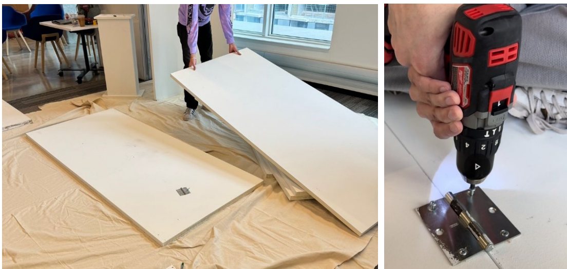
Image 35: Pictures showing assembly of the wall panels as designed.
