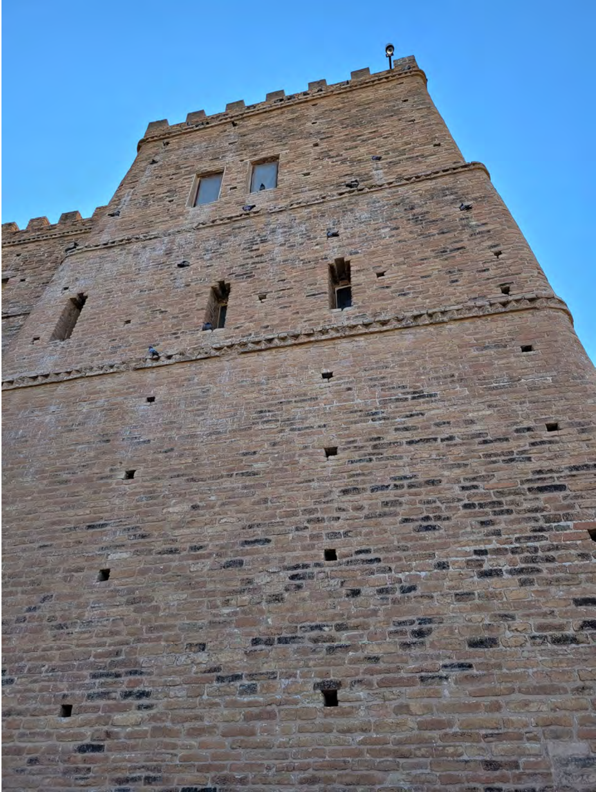
Shush Castle (Château de Suse), built late 1890s. Photo Credit: Abedar Kamgari, 2022.
