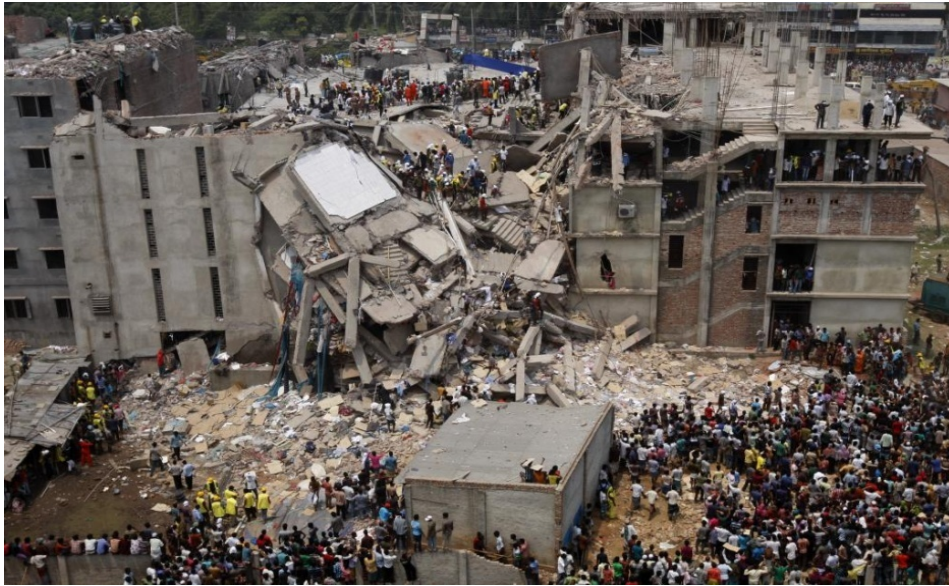
Figure 4: Site of the Rana Plaza accident on April 24, 2013 (Source: Daily Star, June 04, 2015)
