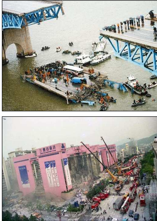
Figures 7a (top). Collapse of the Söngsu Bridge (1994). Source: Yonhap News Agency. Figure 7b (bottom). Collapse of the Samp'ung store (1995). Source: Yonhap News Agency.
