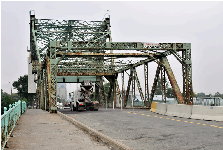
Fig.41 Cherry St bascule bridge with Warren truss
