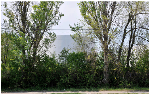
Fig.28 Oil tank farm
