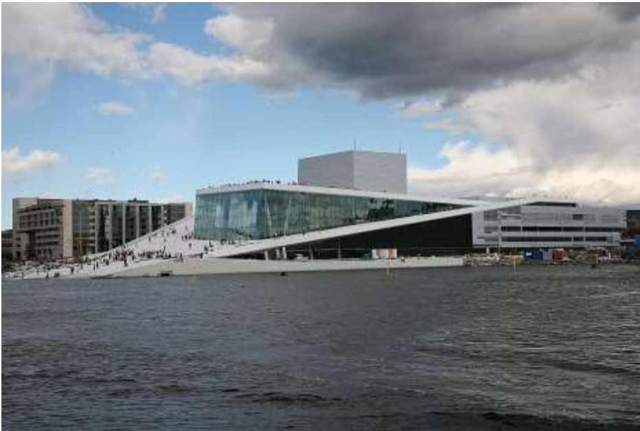
Figure 3: An example of the continuous surface is the roof of the Oslo Opera House by Snøhetta. The design was from 2000 and the Opera House was finalized in 2008 (Photo: Hans Rosbach 2007, Gnu free documentation license).
