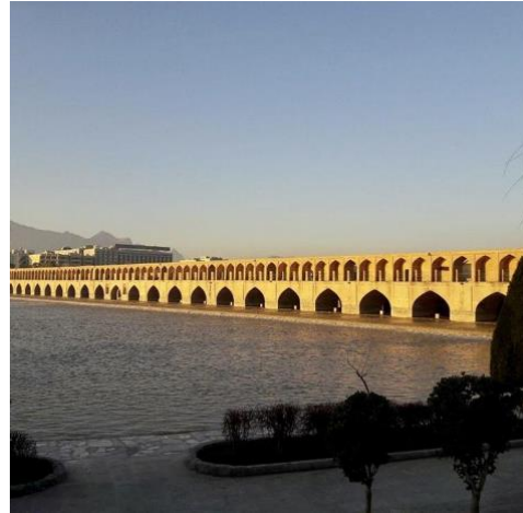
Fig. 3. “Allah Verdikhan Bridge”. Isfahan, Iran
