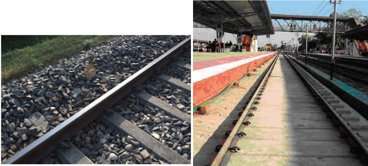
Figure 16. Left: ballast on tracks. Right: Washable apron (source NEFR Railways website)
