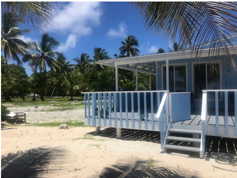
Figure 9. Photograph of house completed in 2019 in Majuro, RMI constructed of PVC pier foundation and wood framed construction. It demonstrates slight innovations in housing design for Majuro.
