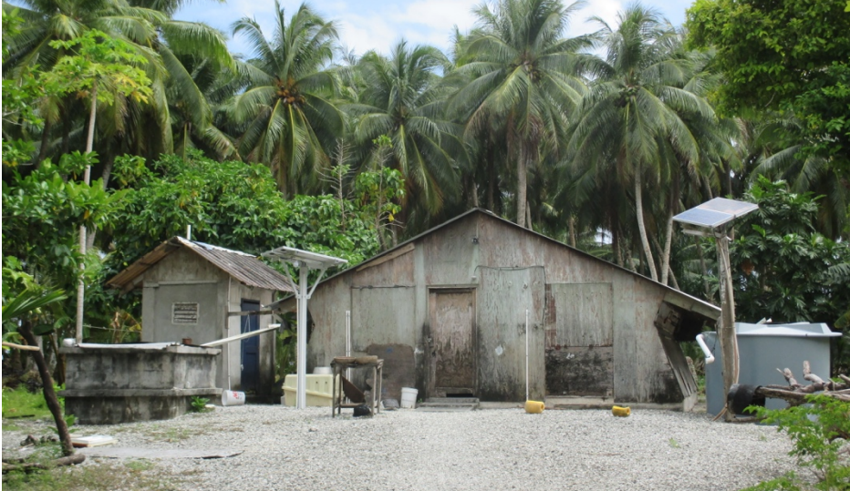
Figure 5. Post-disaster shelter deployed by FEMA after Typhoon Alice devastated Namdrik and Jaluit atolls, RMI. This wood framed structure with concrete slab on grade, is a one room dwelling used primarily for sleeping and crafts making.
